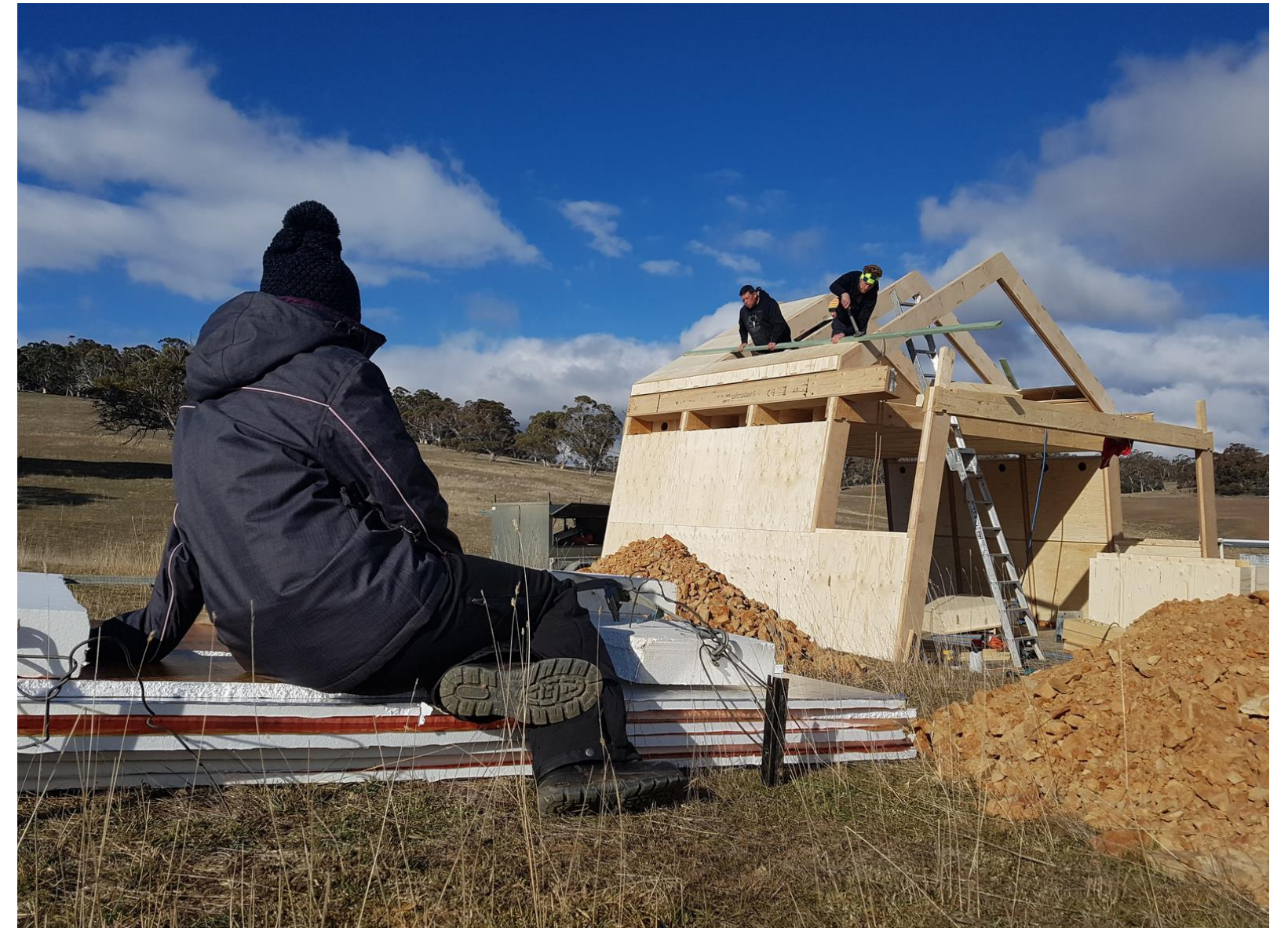
the construction of the prototype ecokit home in 2018 in AU
