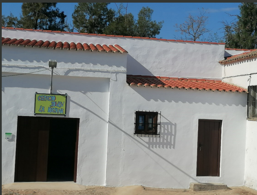
Fachada principal rehabilitada
